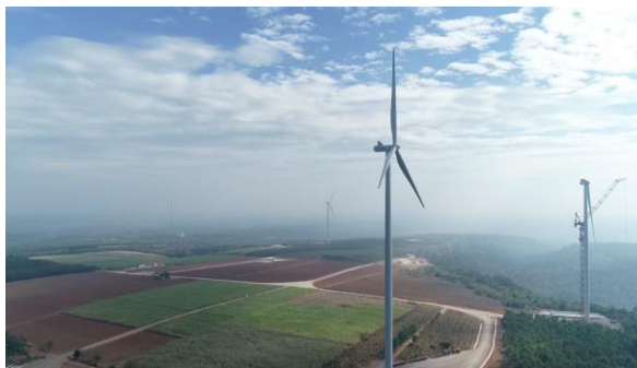
Figure of Romklao Wind Farm
